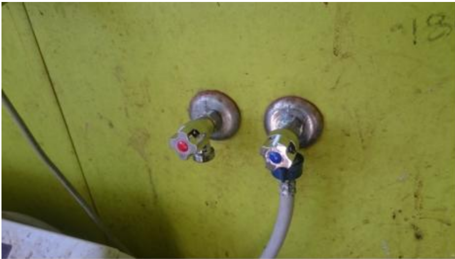
House 16 - leaking washing machine taps replaced
