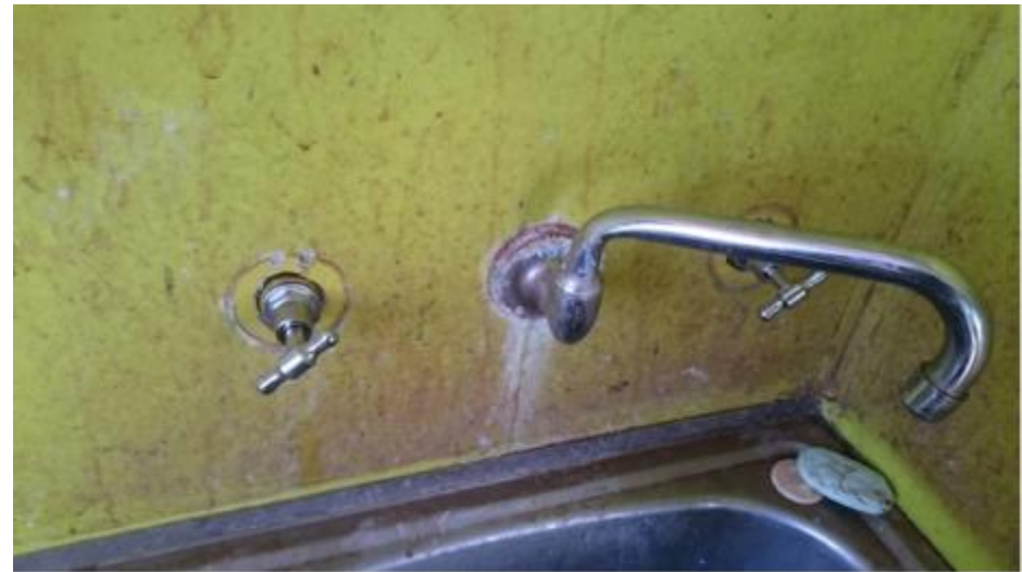
House 16 - leaking laundry taps reseated and spindles replaced
