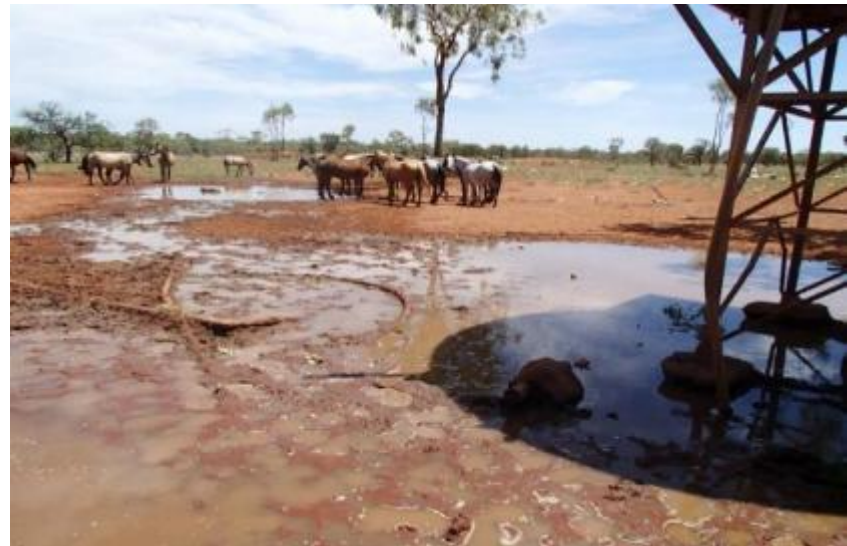
Plumbing Damage from Feral Animals
