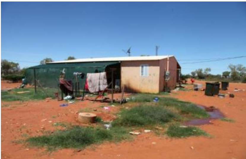
Damage from cars and foreign objects
